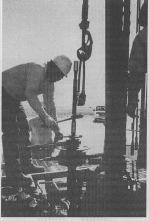
DOWNHOLE DATA — An oil well worker installs a downhole dynamometer on a sucker rod string during a field test in 1996. Data from tests at six producing US oil wells are included on a Sandia CD-ROM available free to members of the oil industry.
